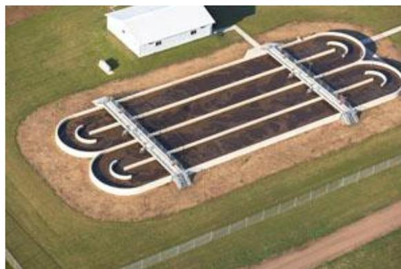
Figure 2. Oxidation Ditch
